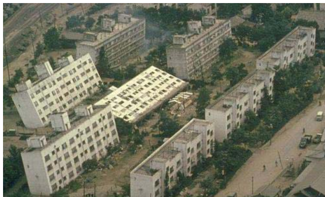
Effects of soil liquefaction from the Niigata earthquake, 1964, (from Earthquake Engineering Research Center Library, University of California at Berkeley).
